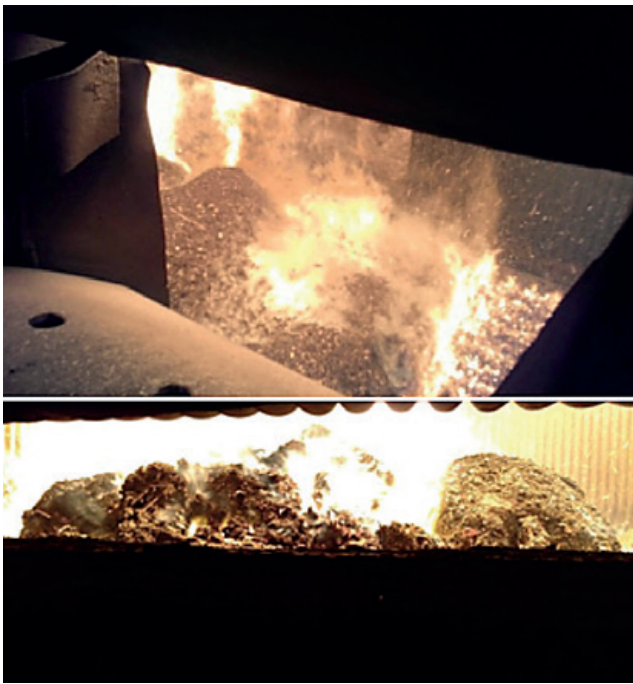
Figure 12. Photos of the layer of material on the grid accumulated by bad combustion
