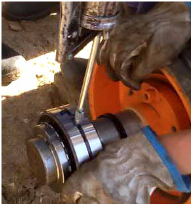
Figure 8. Grease added inside the sealed bearing
